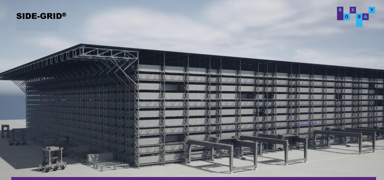
The Side-Grid has interfaces on both the end faces and the longitudinal sides. Because trucks are serviced via CPC loops and Truck Transfer Cranes on the longitudinal sides, it is called the Side-Grid.
