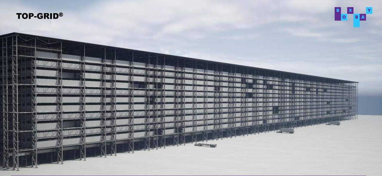
In the Top-Grid, the warehouse is elevated and accessible from below. AGVs or automated trucks operate at ground level beneath the aisles and are serviced directly by the Stacker Cranes from above
