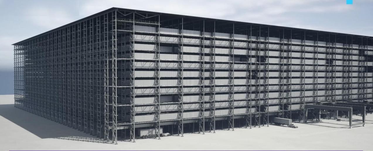
The Hybrid-Grid combines features of both the Top-Grid and Side-Grid. AGVs or automated terminal trucks are serviced direct under the HBS, landside truck traffic is handled using CPC loops and truck cranes.
